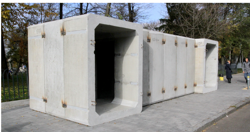
Figure 23. The photo of the temporary modular bomb shelter structure in Dnipro.
