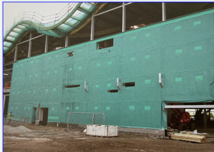
Joonis 24: Hemclad® paneelide paigaldus (The Hempcrete Book)
